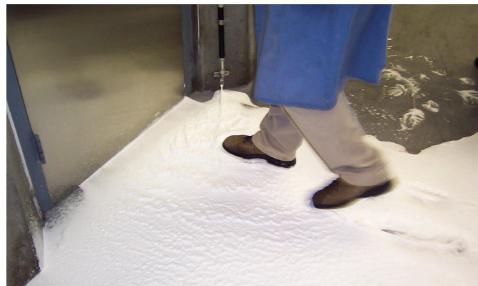
Doorway Foam Units
